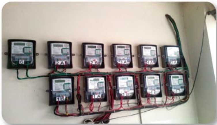
Replacement of Conventional Meter by Pre-Payment Meter
