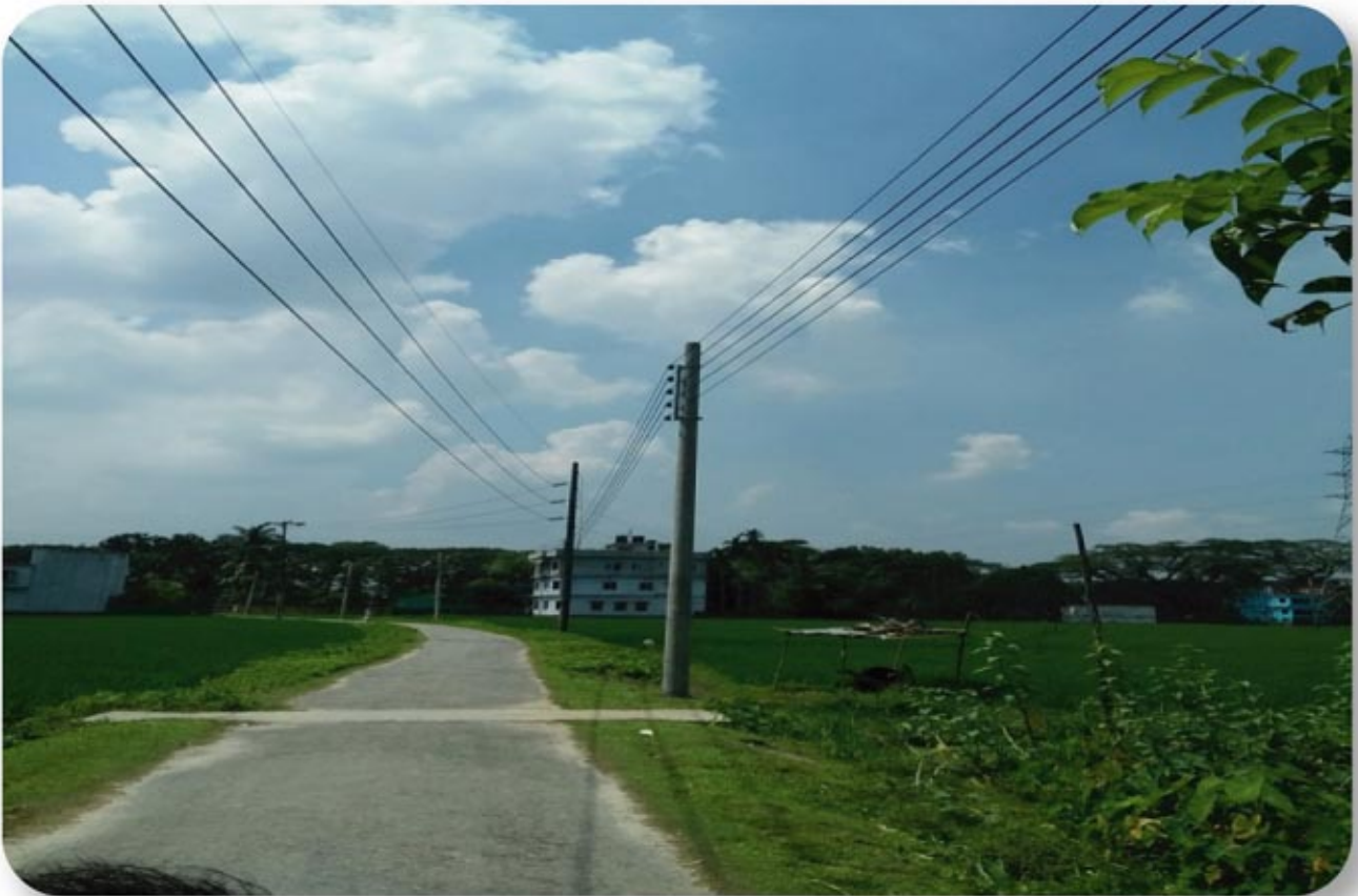
Newly Constructed Distribution Line at Jinaidah
