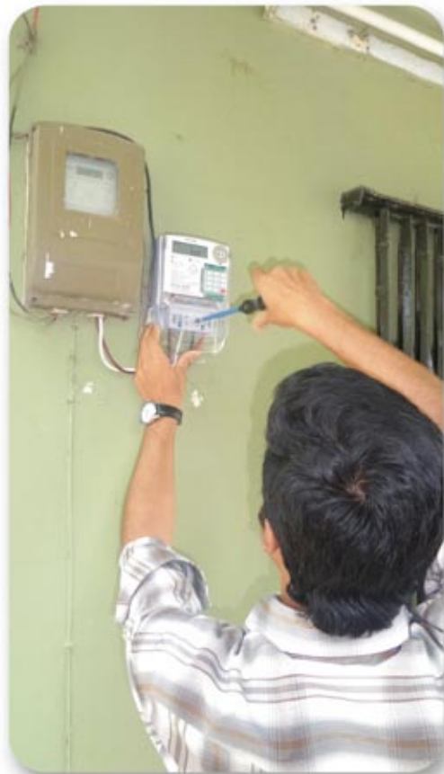
Replacement of Conventional Meter by Pre-Payment Meter
