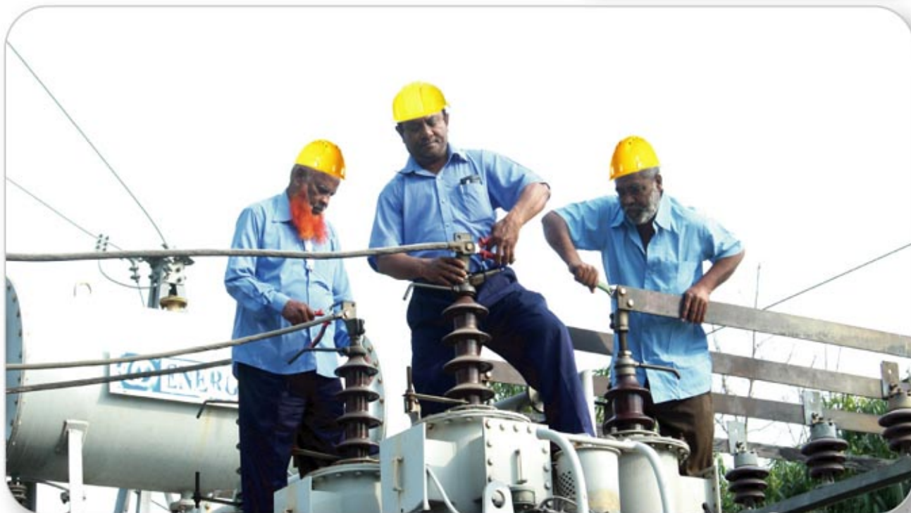
Scheduled maintenance work of 33/11 kV Substation
